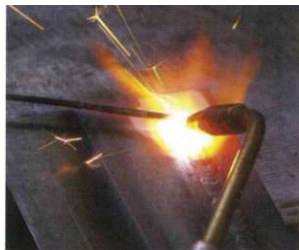
Gas welding using oxyacetylene
